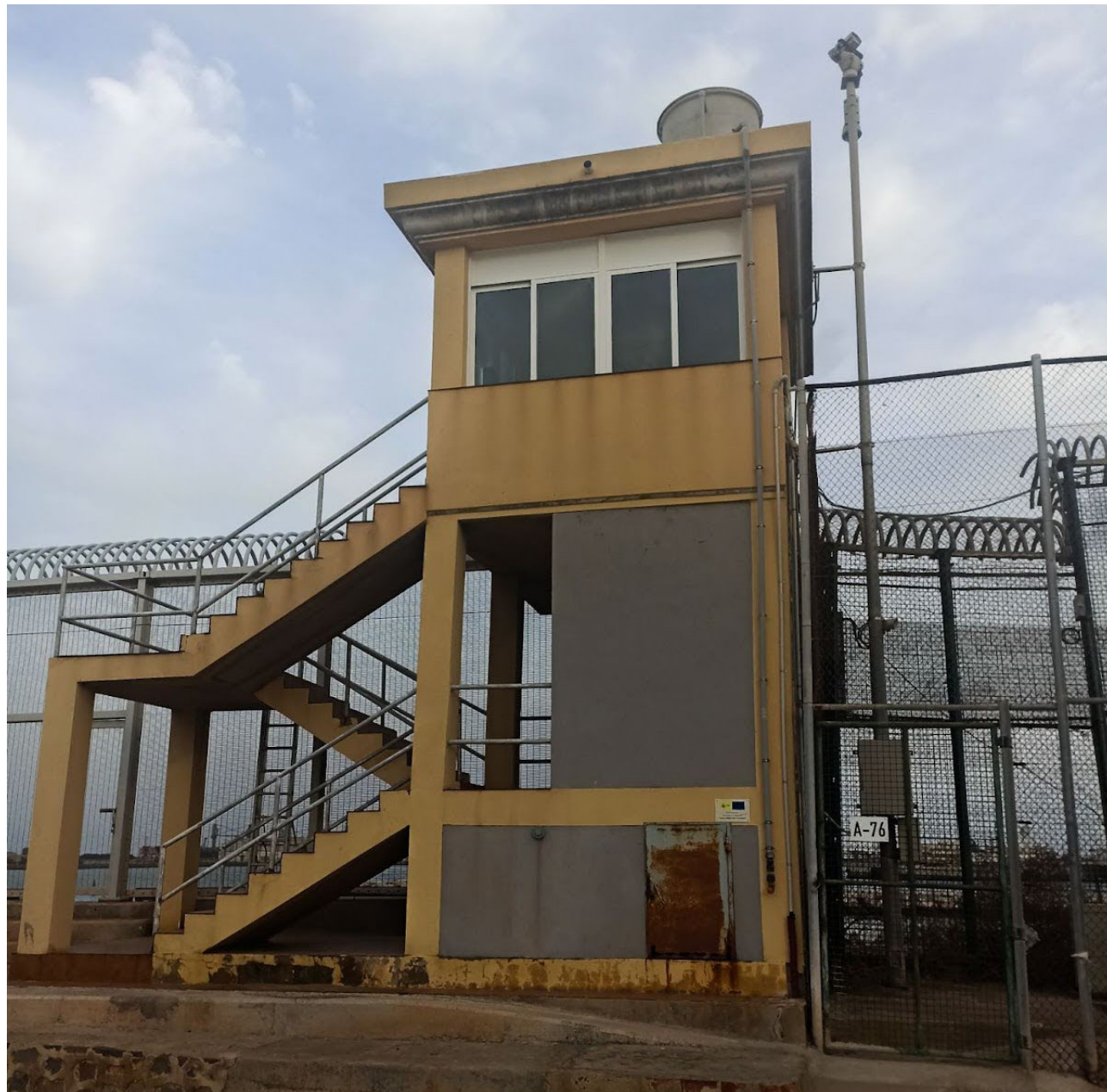
Figure G: Carlos Lancho. A surveillance tower near the Paseo Marítimo, in Melilla.
