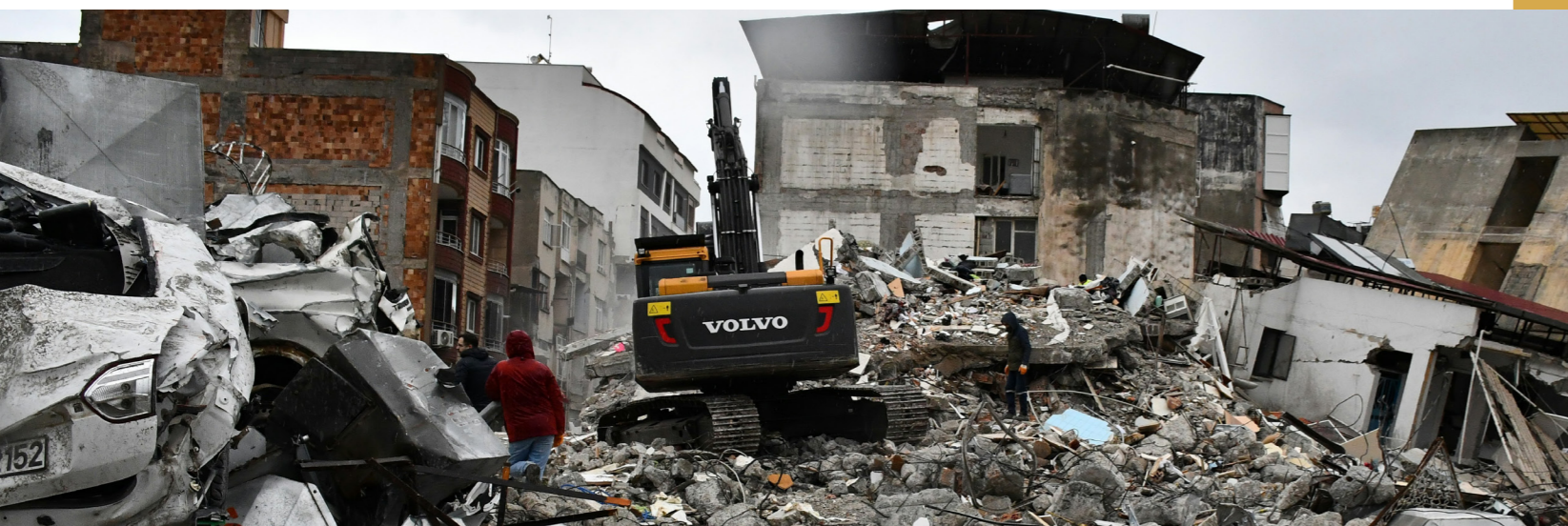
© Çağlar Oskay - Iskenderun, Hatay Turkey - February 2023: In Iskenderun, one of the places most affected by the 7.7 magnitude earthquake centered in Kahramanmaraş
