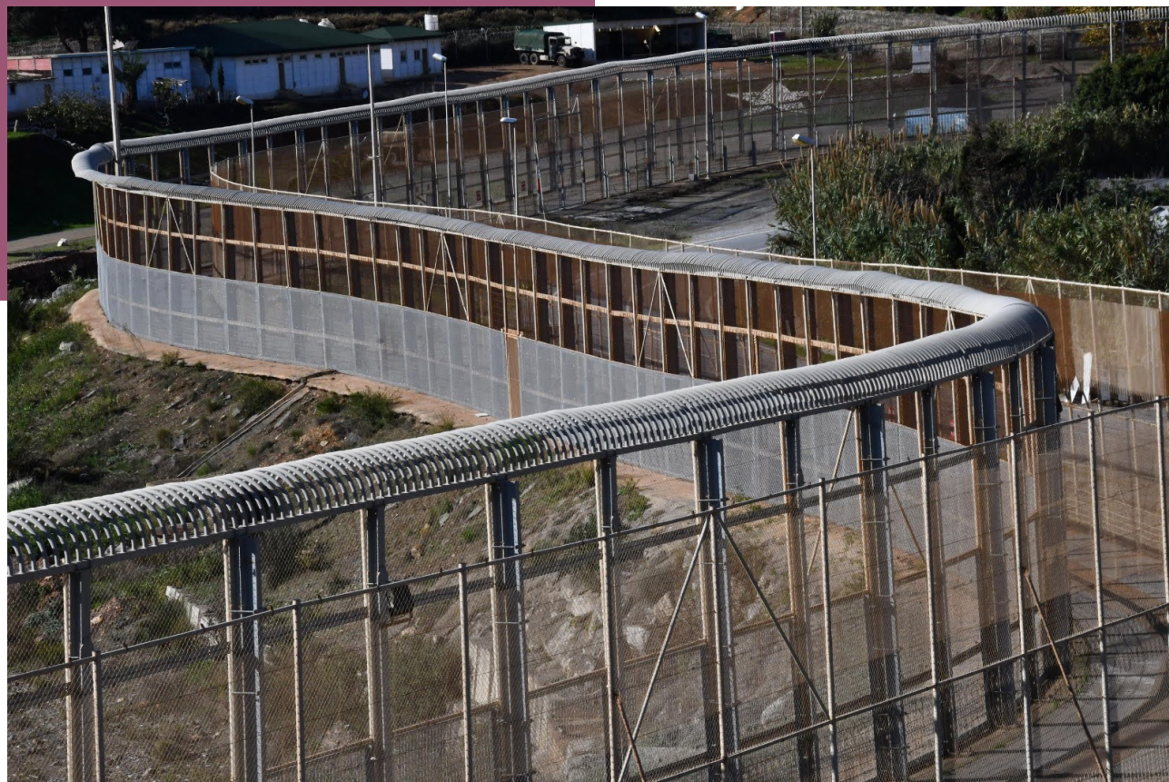
Figure D: El Faro de Ceuta. A bird's eye view of the Ceuta fence showing the inverted combs.
