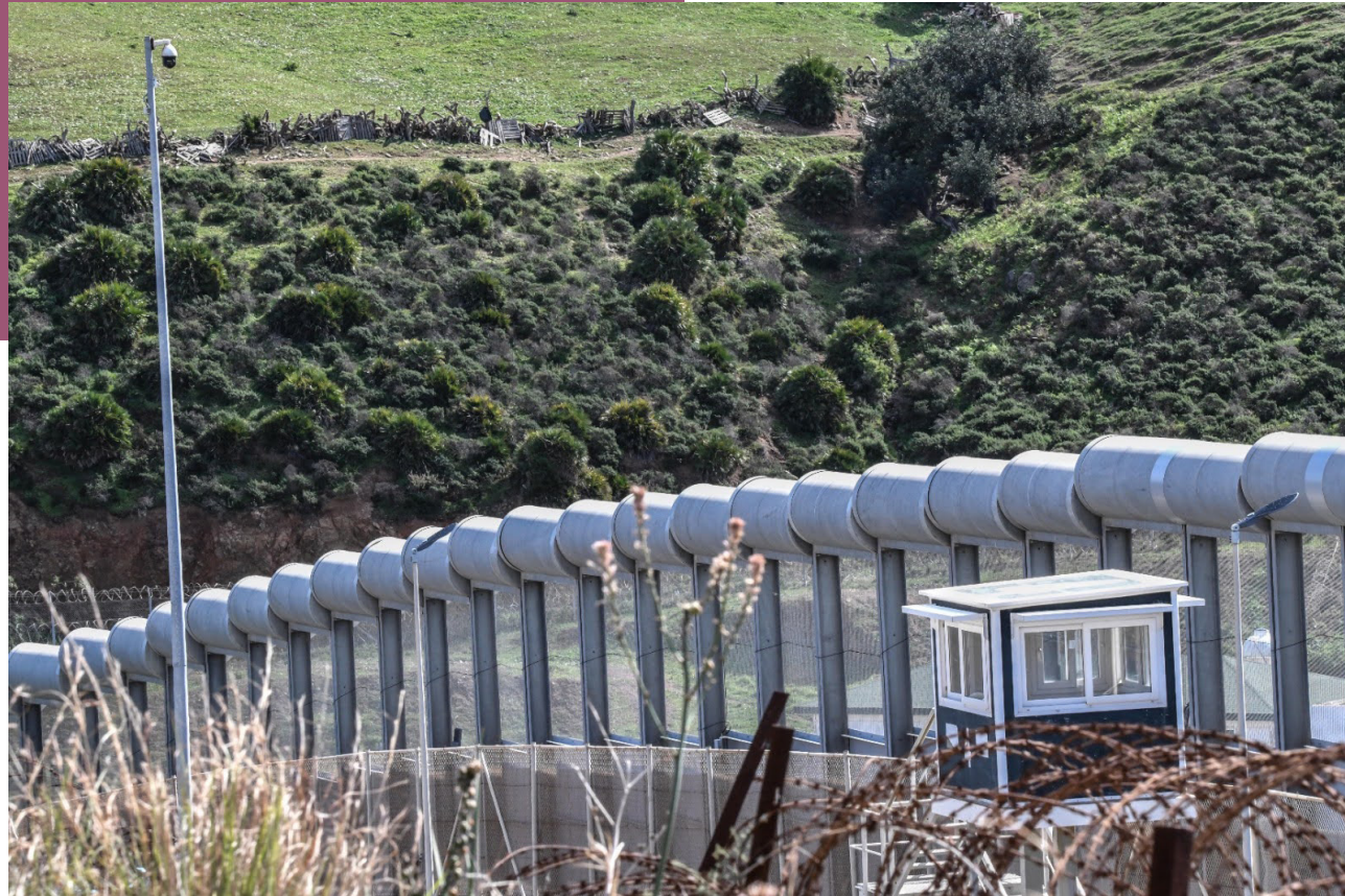
Figure F: El Faro de Ceuta. The new prototype of the Ceuta fence showing the anti-climbing cylinders.
